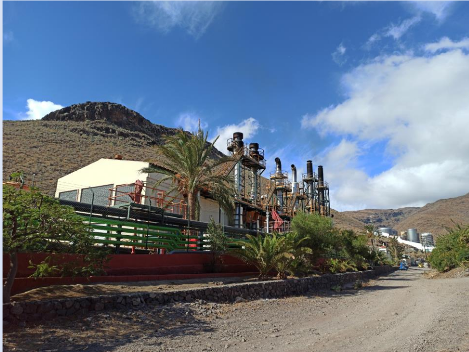
Figure 1: Thermal power plant El Palmar in La Gomera © HATECHNO
